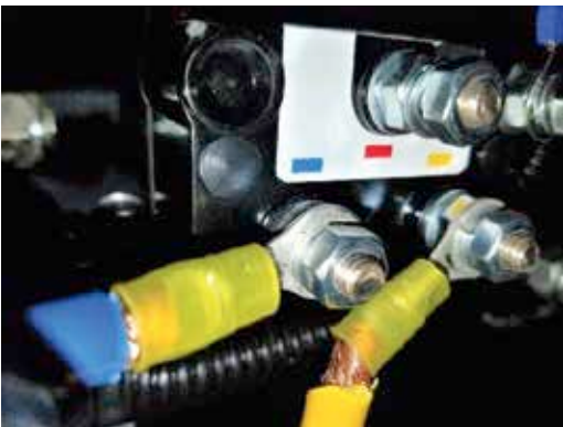
Figure 9: Electric Cables to Controller
