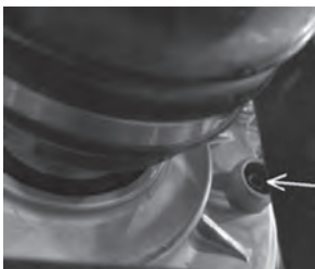
Front Differential Check/Fill plug
