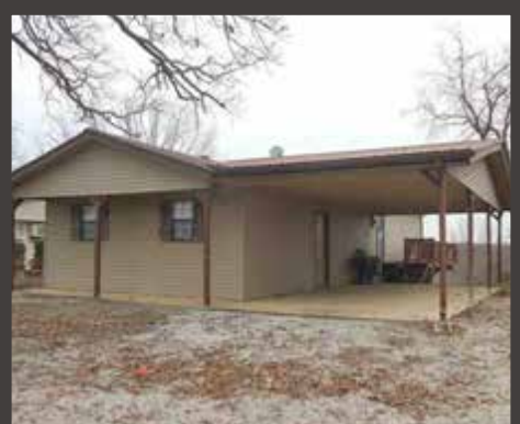
Lake Life is Great! 3 bedrooms, 1 bath, great room. Furnished! Remodeled, neat and clean, large deck, lake view, boat slip! Turn key Fun! Partial basement, has garage for ATV. You can literally walk to hunting or lake. $115,000 #116279
