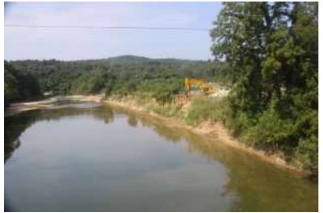
Figure 1. Severely Eroded Bank Before Construction-July 2010
