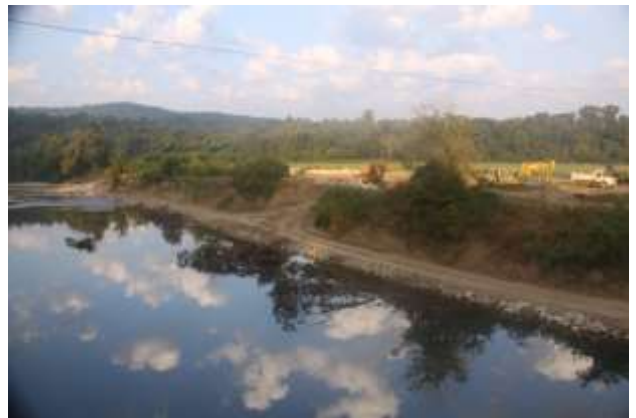
Figure 2. Same Bank During Construction-July 2010
